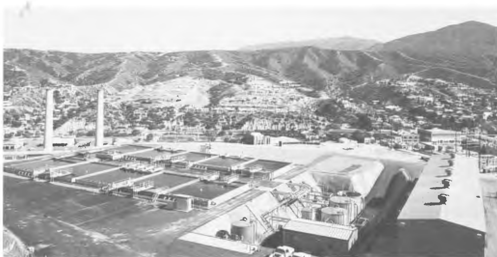
An example of a modern solvent extraction-electrowinning facility is this Cities Service Company's installation at Miami, Arizona. It was designed and constructed by Holmes & Narver, Inc., Orange, California, to produce 30,000 pounds of cathode copper daily. (Ray Manley photo courtesy of Holmes & Narver)
