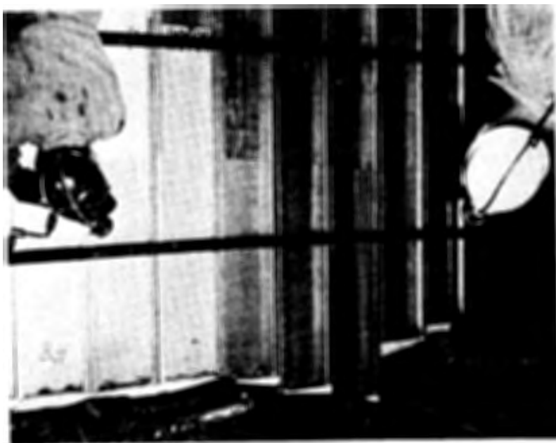
FIG. 58 INSTALLATION OF METAL STOPPING PANELS
