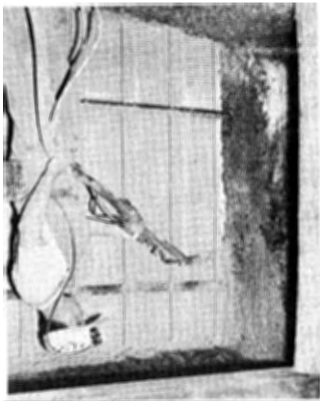
FIG. 58 INSTALLATION OF METAL STOPPING PANELS
