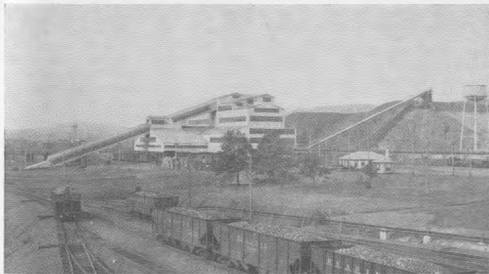
A modern mineral preparation plant in the anthracite field of Pennsylvania. In a yearly period this plant will prepare for the domestic heating market 2.5 million or more tons of anthracite in as many as 12 different sizes.
