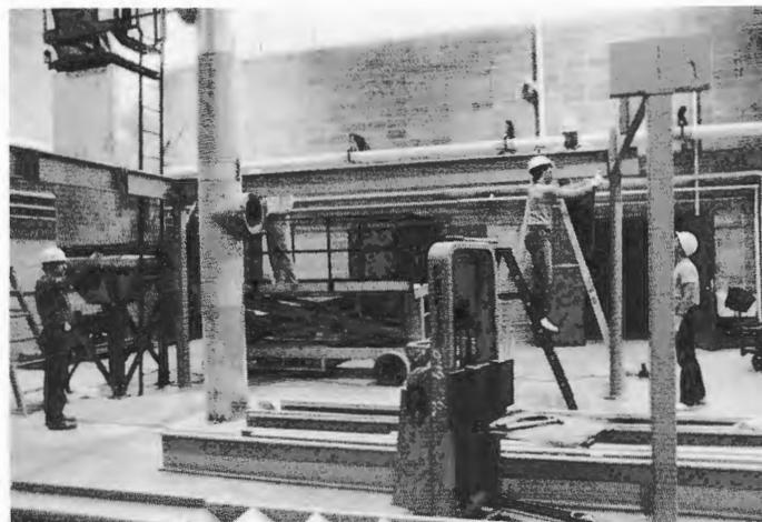
Figure 1. Installing the support structure for the research boiler in the new Combustion Laboratory.
