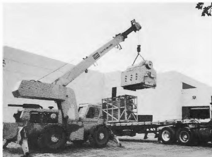
Figure 2. The research boiler is unloaded prior to installation in the Combustion Laboratory in Penn State's Academic Activities Building, seen in the rear.
